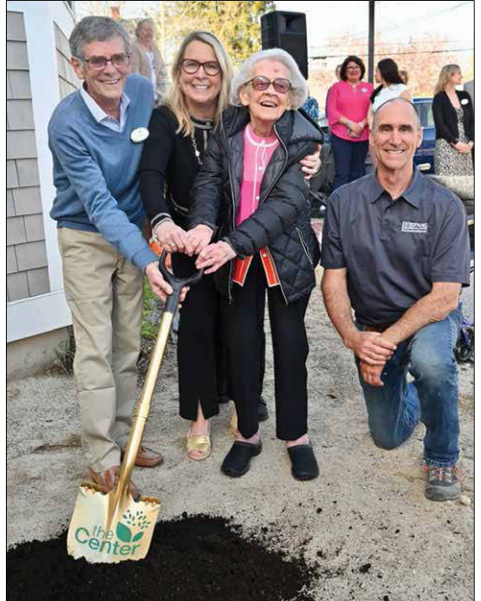
Groundbreaking crew (L-R): Capital Campaign Chair Andy Spaulding, Executive Director Bridget Dempsey, founder Annie Spaulding and builder Tim Spang. Photo by Bob Dennis
